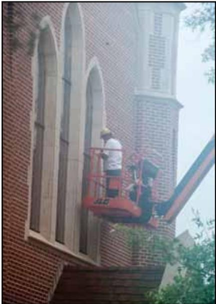
continuous effort, workers completed the painstaking process of restoring the exterior surfaces of the Abbey Church. The work process included replacing mortar joints, repairing masonry, cleaning brickwork and waterproofing the surfaces. The result is a very noticeable improvement in the appearance of the church and will go a long way in preserving it for years to come. This work was made possible through the generous donations from some 154 donors.
