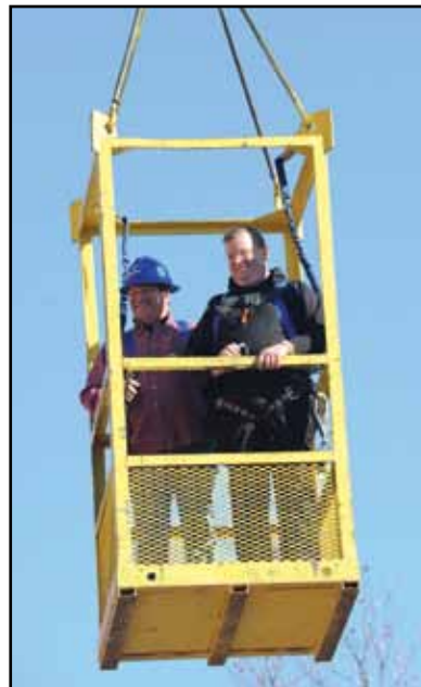
At far left – photos show the damage and demolition of one of the turrets of Benedictine Hall that did not collapse during the initial earthquake on Nov. 5. Left – Abbot Lawrence makes a personal inspection of the demolition work from the 150 ft. high view of the construction crane.
